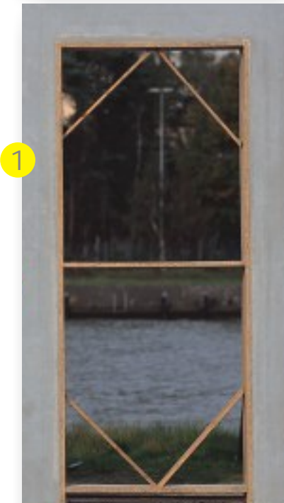
Doorway with formwork. Any sizes are possible.
