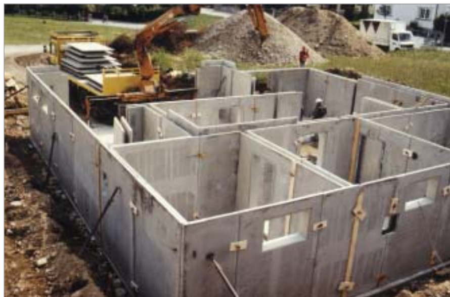
A residential building being assembled from prefabricated double walls. The next step is the installation of the wall elements, which are also prefabricated
