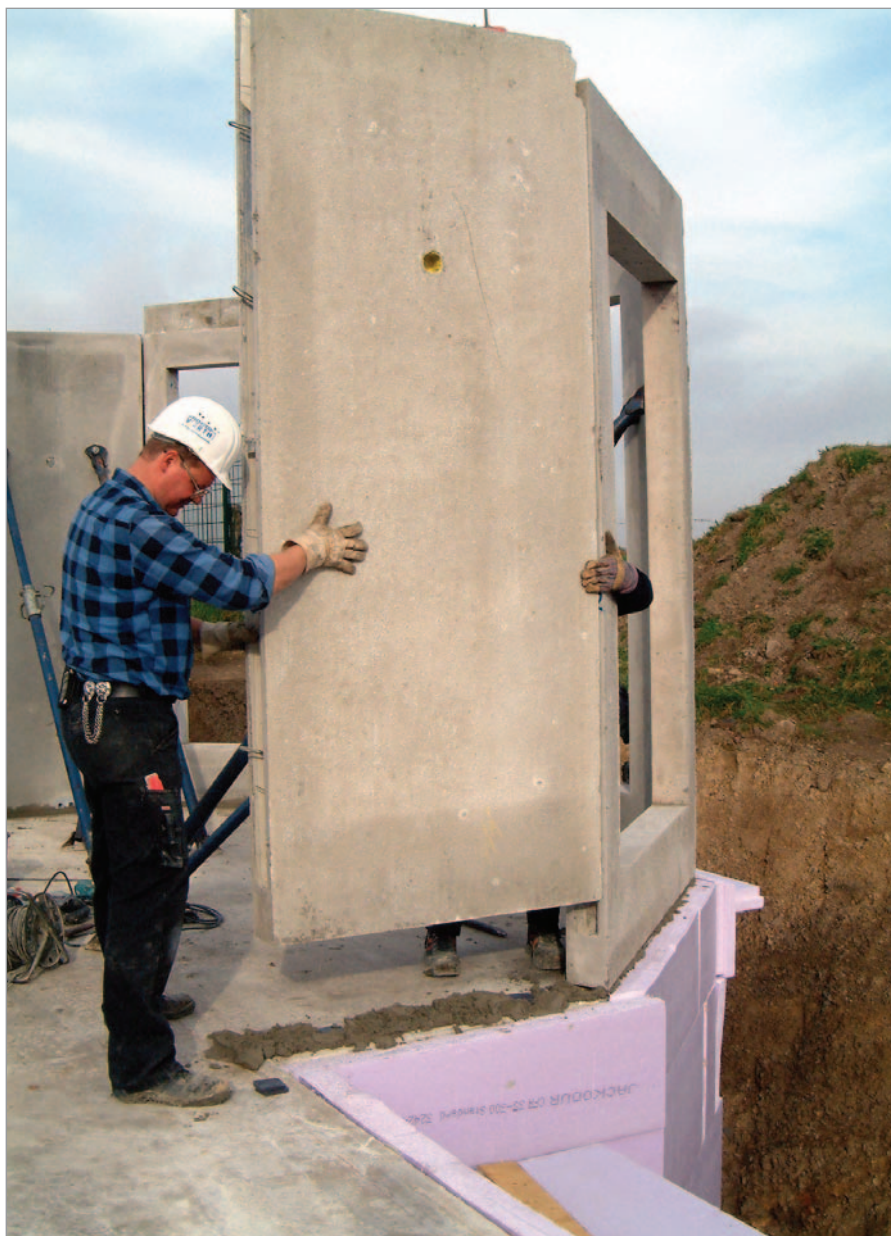
The use of high quality building materials and systems complements the short assembly time for the precast units made of concrete and lightweight concrete, creating an economical, forward looking method of building
