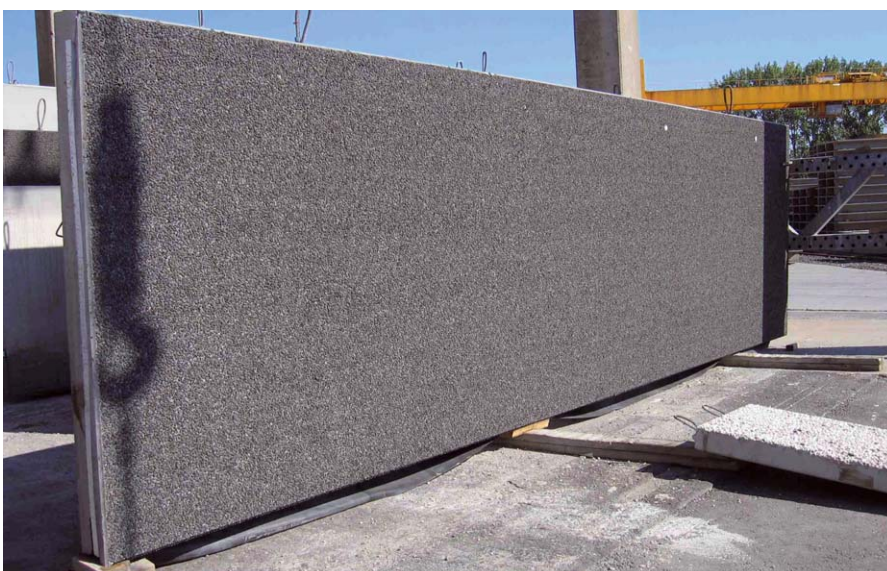
Facade elements with washed concrete surface and integrated thermal insulation
