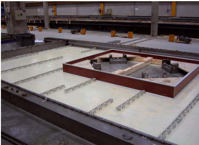
Pallet fitted with formwork with window recesses
