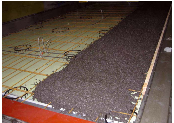
Concreting the exterior shell
