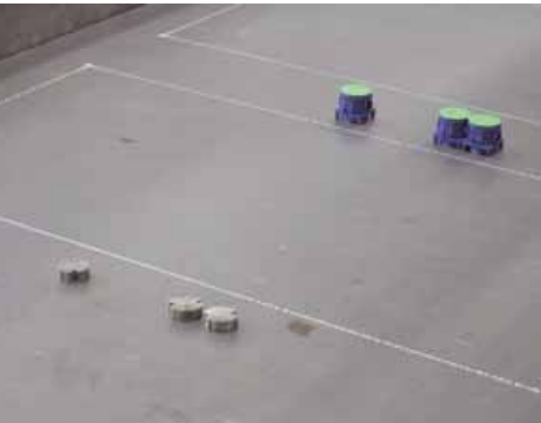
Electrical back box magnets ensure the exact position of the back boxes for switches
