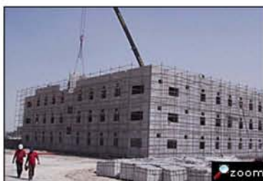
Labour housing in Al Warsan, Dubai.
