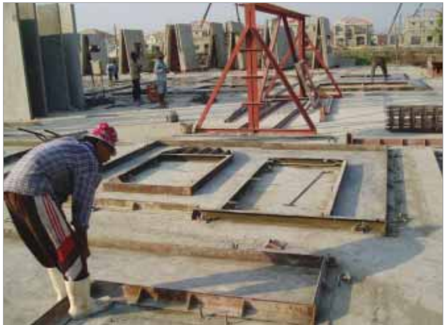
Preuksa casting yard
