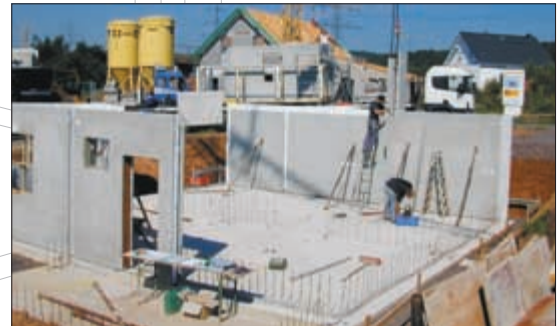
Basement construction with prefabricated SysproPART thermo wall elements
