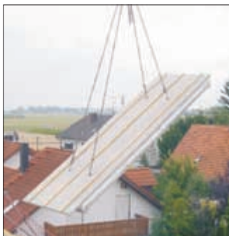
Mounting a Syspro thermo roof
