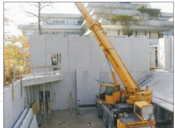
Mounting of 10 m high SysproPART thermo wall elements at Ulm University
