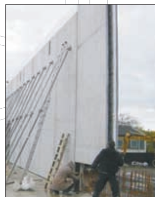
Mounting of 10 m high SysproPART thermo wall elements at Ulm University
